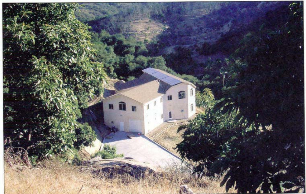
Ellsworth's solar-powered, green-built facility was constructed in an abandoned avocado grove in southern California. Recent wild-fires destroyed the avocado grove but the factory was saved, due in part to its polysteel cement structure.
